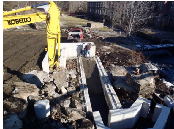
The construction of a steep pass fishway around the Hallville Dam (Poquetanuck Brook, Preston) back in December. This fishway is now completed and will be passing fish soon. More in future reports.
